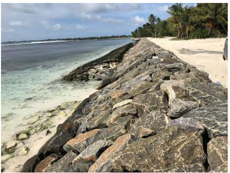
Figure 5. Rock Revetment Example
