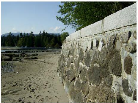
Figure 9. CRM Seawall Example
