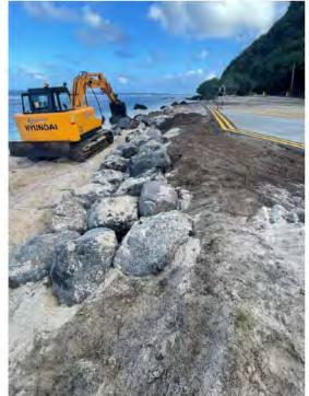
Photo 9. View to the northeast showing heavy machinery working in shoreline protection project area, moving rocks and dirt to repair damage done by king tides and to protect airfield.
