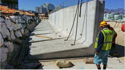
Figure 11. Precast Concrete Seawall Example
