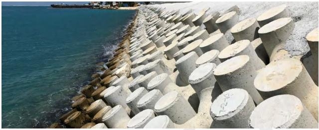
Figure 7. Tribar Revetment Example
